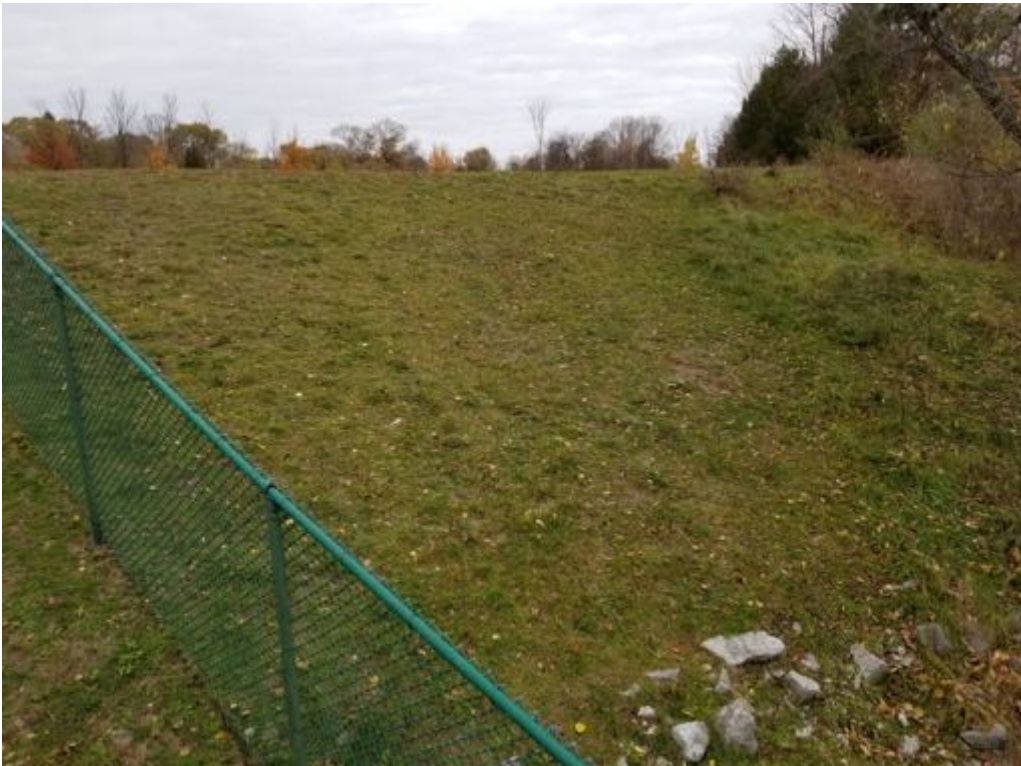
Downstream embankment at east end
