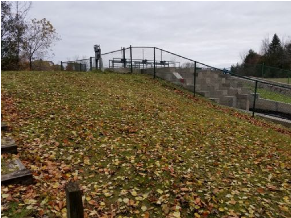
Downstream embankment west end of dam
